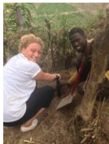
Digging fence post foundations
