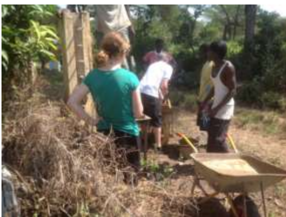
Lloyds Group help construct new fence
