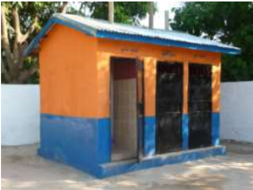
New pre-school toilets
